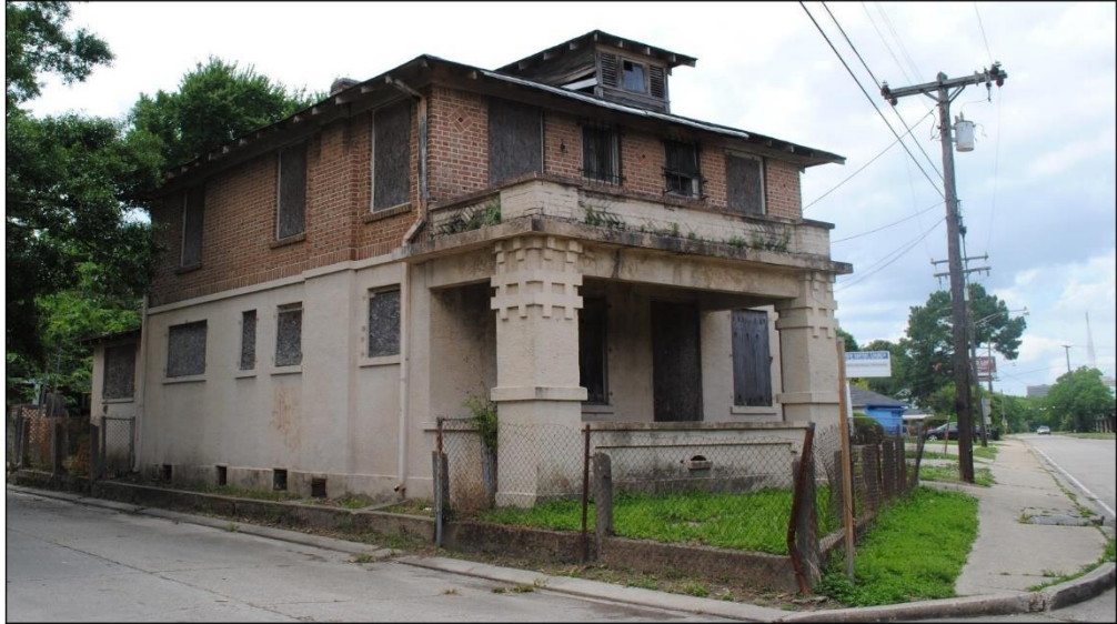
Photo 10 1666 Braddock St. at the corner of Lettsworth St. and Braddock St. (17-02057)
