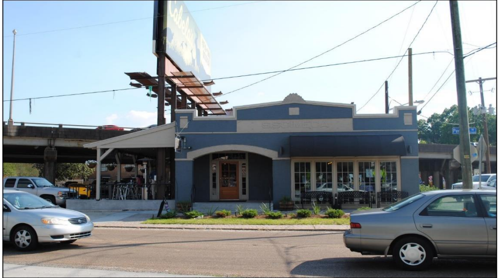
Photo 17 Overpass Merchant at 2904 Perkins Rd. (17-01920)
